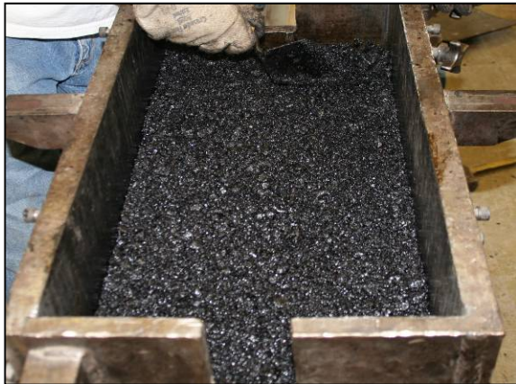
(a) Leveling of Mix in LAC
