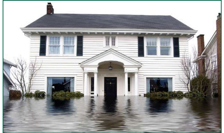
Water damage to homes from hurricanes and floods can be excessive. Mold and pollutant contamination have a lingering influence after these disasters that impedes the health and the return of the homeowners to their dwelling.
