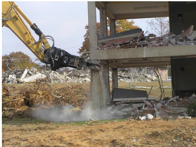
(b) corner column removal in field test Hinge Zone
