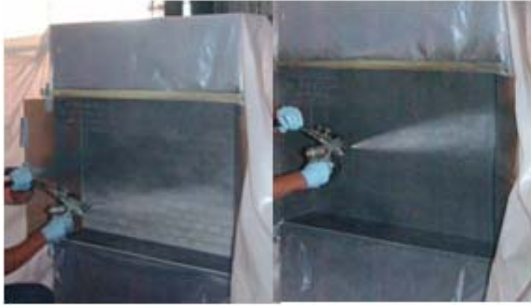
Figure 22: Spray-on retrofitted material
