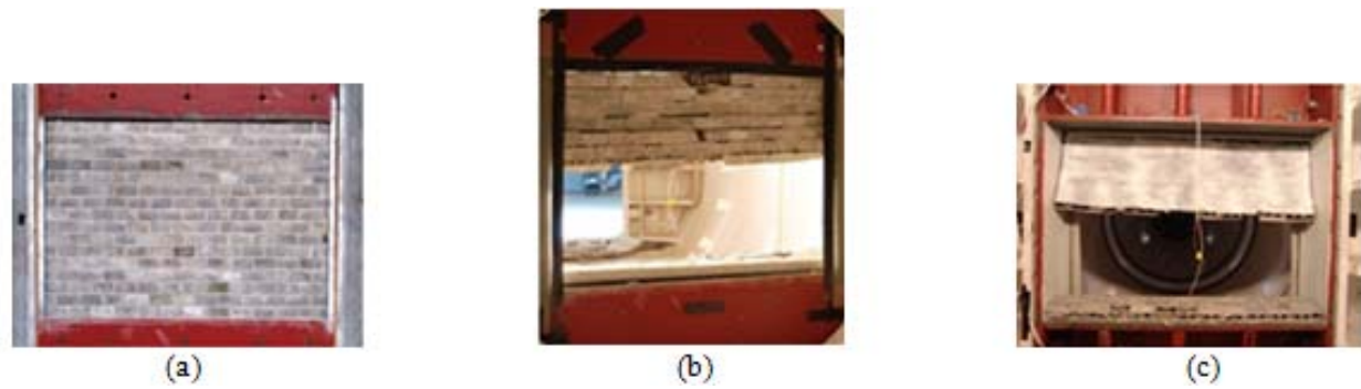
Figure 26: Wall #2 (a) front view before the blast event (b) front view after the blast event (c) back view after the blast event
