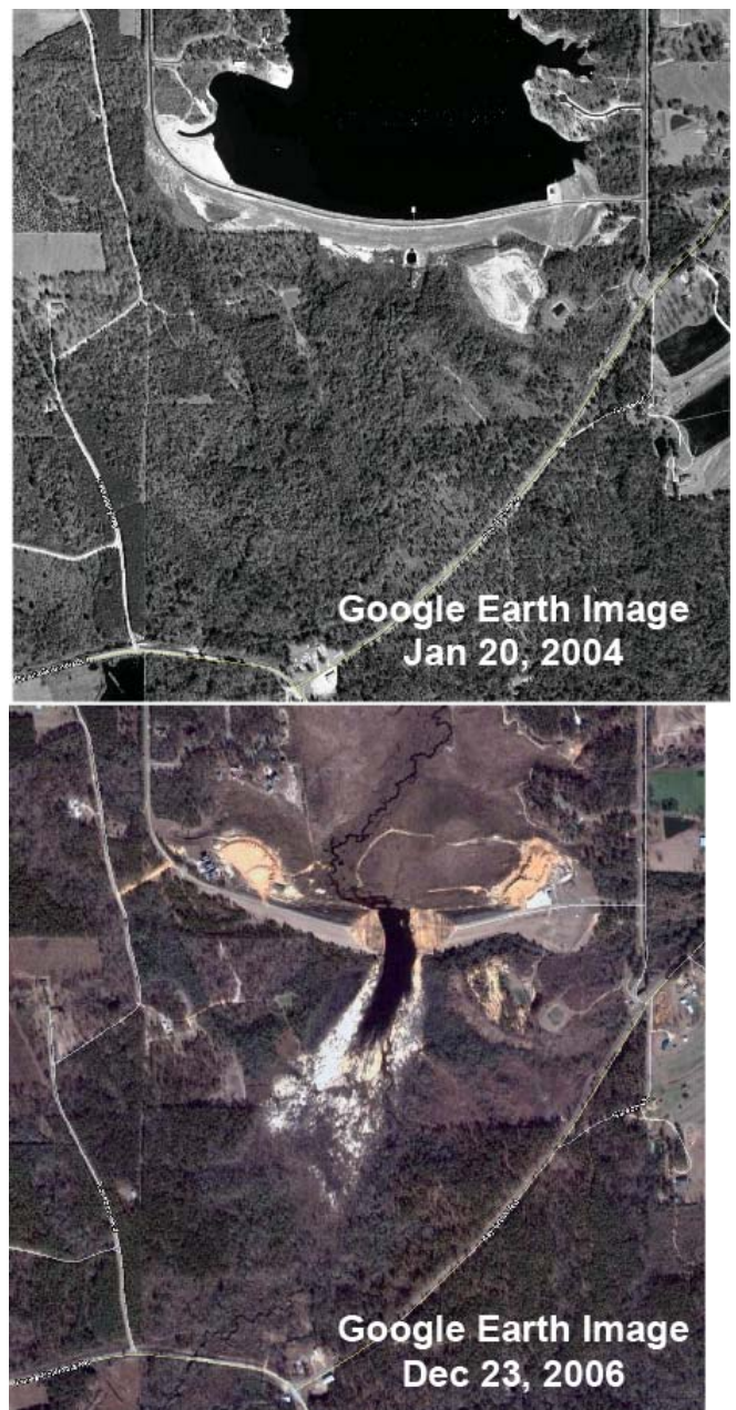
Figure 1. Satellite images of the Big Bay Dam before and after the failure. The scar left by the flood waters is clearly visible in the image below.
