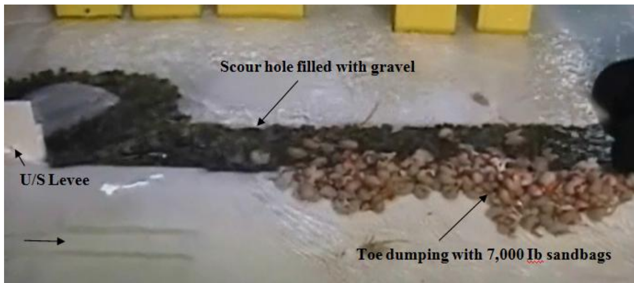
Fig. 4.5. Toe dumping of 7,000 Ib sandbag starting from the embankment
