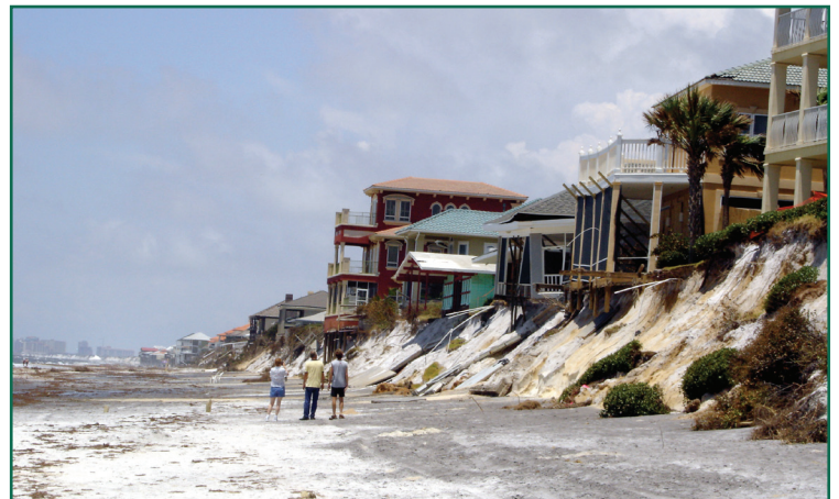
Storm-induced erosion, such as that pictured at Walton County Beach in Florida, has had a dramatic impact in the country's coastal regions. The research team will investigate the effectiveness of wetland vegetation in mitigating wave and surge impact in these areas.
