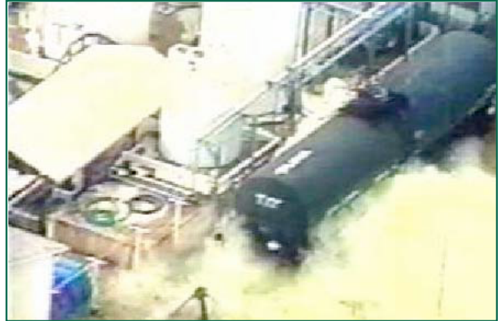
Example of a TIH Material Leak.
