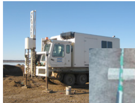
Visual Inspection Ground Geophysics
