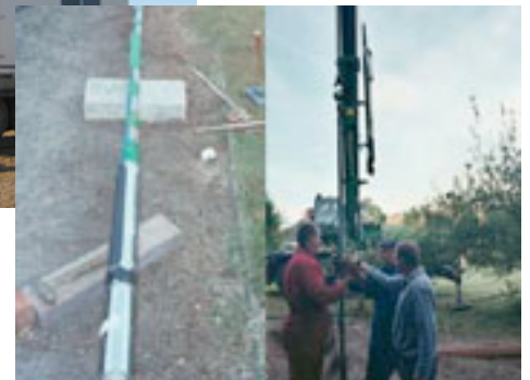
Cone Penetrometer Coring Instrumented Boreholes Trenching
